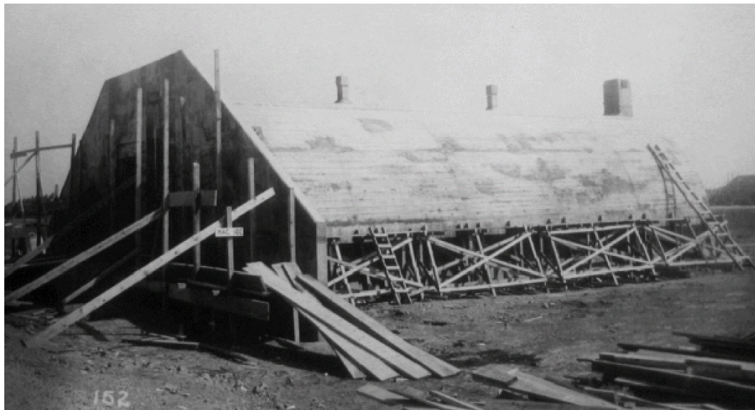
Magazine under construction. Concrete front wall and vault in place, to be covered with several feet of earth, to the top of the vents on the roof.
