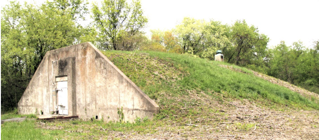
Earth-covered concrete magazine, used to safely store explosives in wooden boxes before being shipped to munitions manufacturing facilities.
